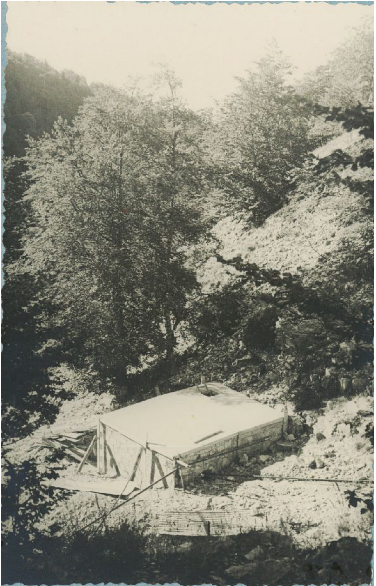
Station de Pompage
